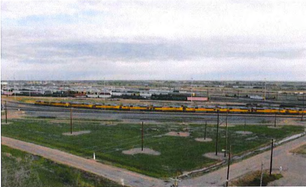
View of Bailey Yard from the Tower
